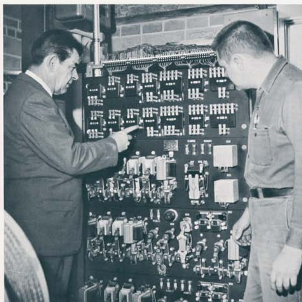
Henry Kieckhefer, Erection Superintendent, and Dave Johnson, Service Mechanic, inspect Anderson selective-collective controller in- stallation.
